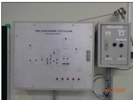
Fire Alarm Graphic Annunciator
